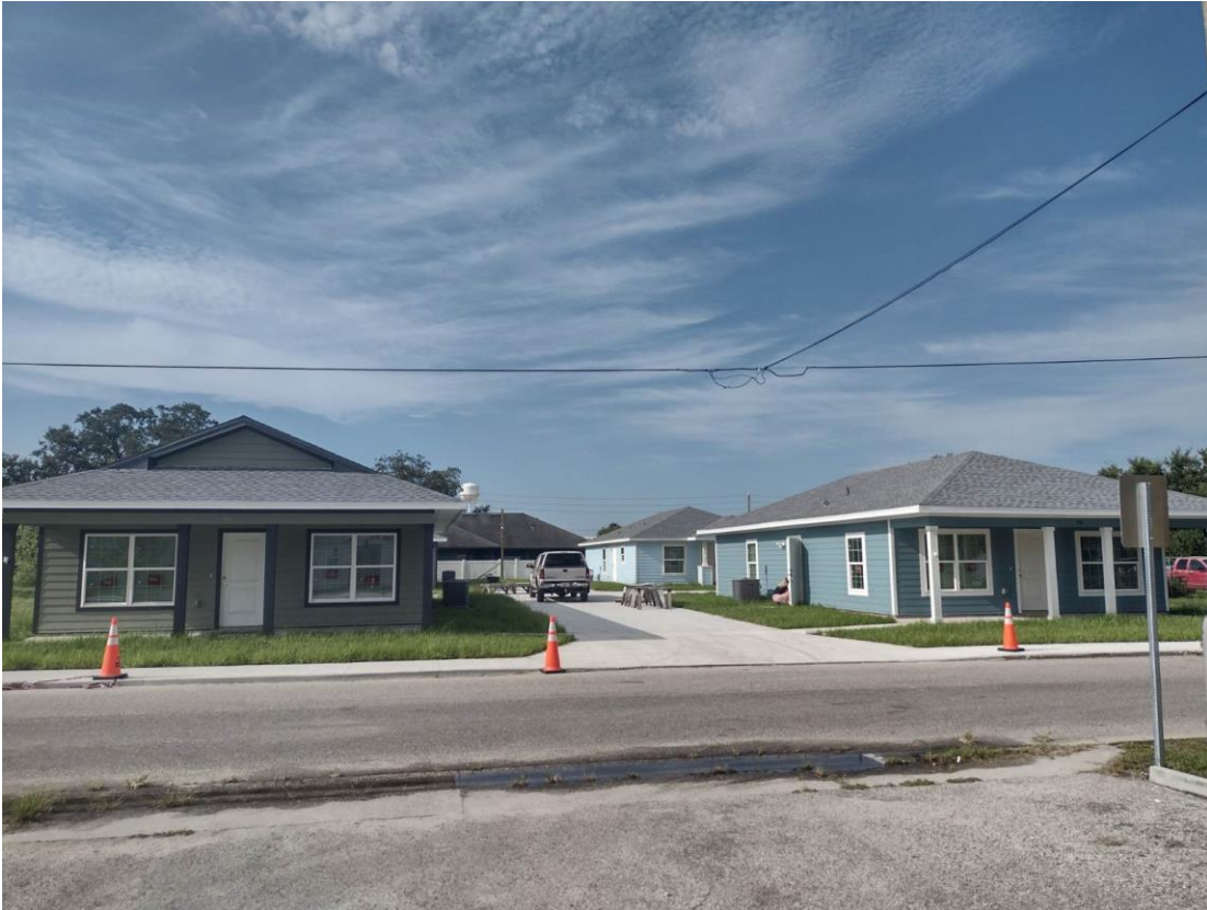
(Facing south towards tandem housing development)
