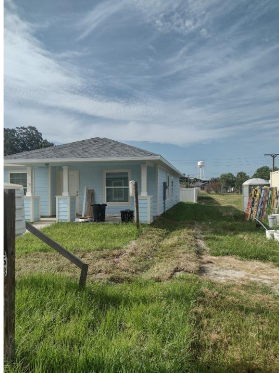
(90 Center Street front and side yard)
