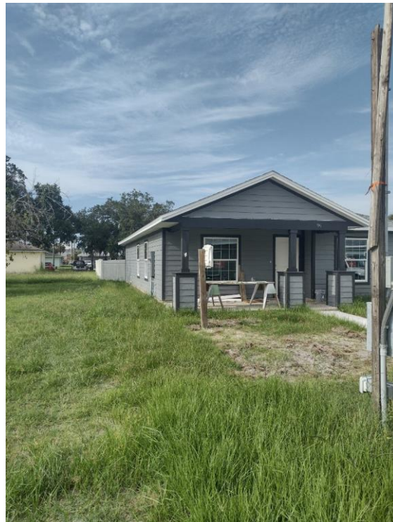
(96 Center Street front and side yard)
