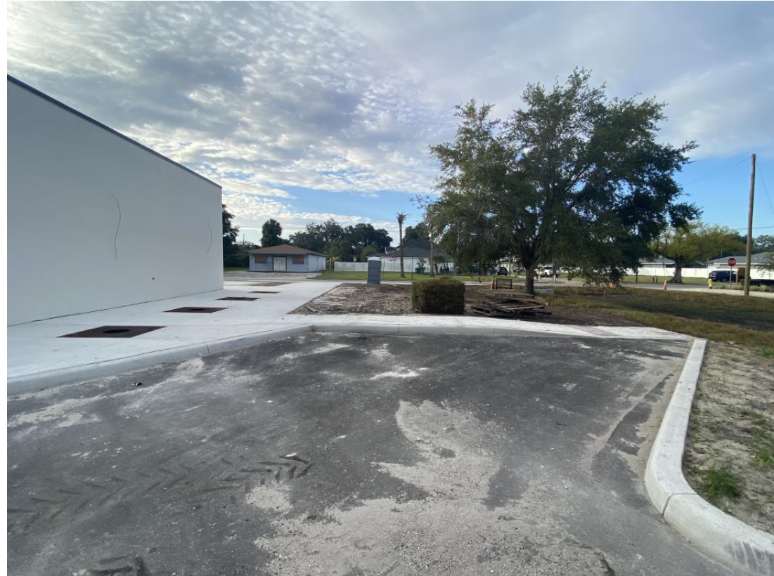
ADA Accessible Parking Area Facing South
