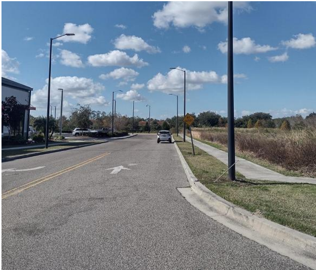
(Facing west along Marcel Drive)
